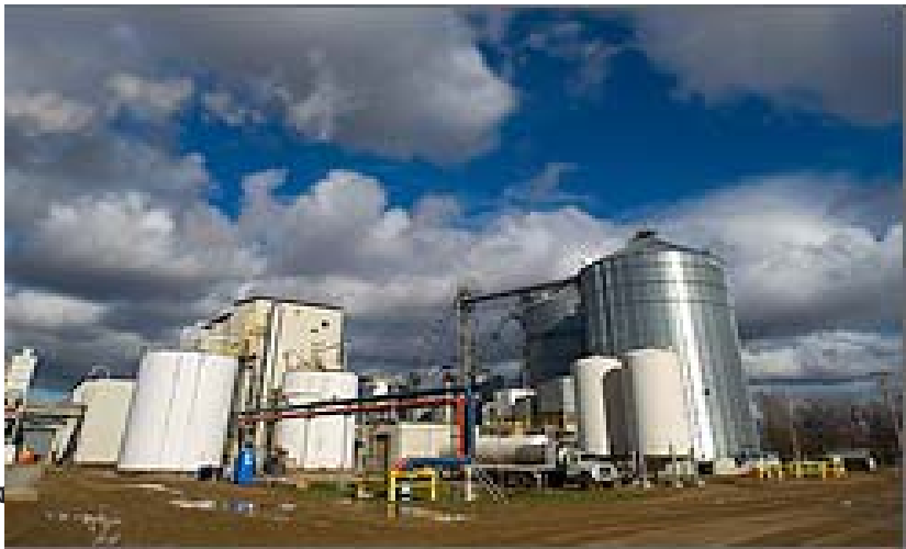
Poet's pilot plant in Scotland, South Dakota, is able to convert corn cobs into cellulosic ethanol at a rate of 20,000 gallons per year.
